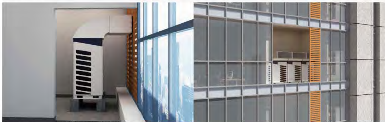
The outdoor unit is hidden inside the building without affecting the overall image of the building
