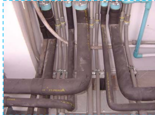
Refrigerant Piping Line
