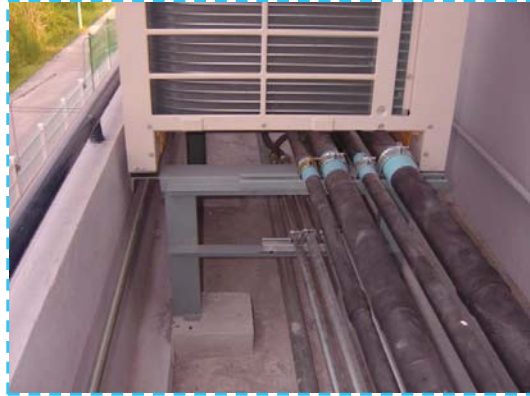
Refrigerant Piping Line
